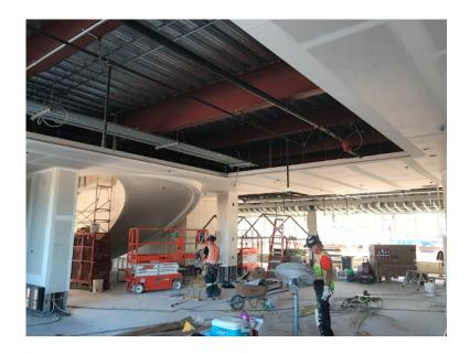
The installation of insulation and drywall is almost complete and ceiling systems are currently being constructed. Windows and storefronts are being installed, the elevator shaft is in place, and exterior scaffolding is erected for surface treatments. The site also continues to take shape with the grading for the new one-acre park, vegetated bioswales, and associated pedestrian bridges
