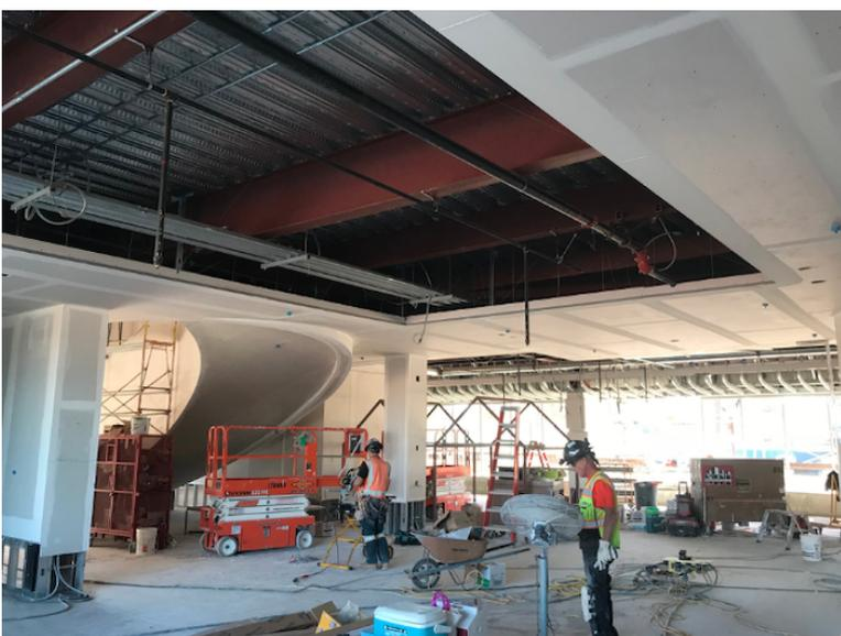
The installation of insulation and drywall is almost complete and ceiling systems are currently being constructed. Windows
