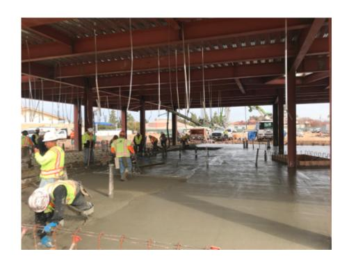
The structural steel frame system for the building has been erected, welded, bolted, inspected, and secured in place. The framework for the large, oval shaped sky light above the future staircase is taking form. The aesthetic arches of the building's exterior are now visible.
