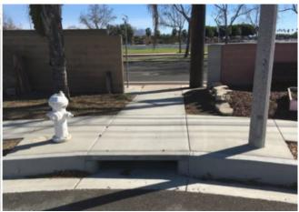
Public Services also recently completed the reconstruction of the parkway drain at Wellesley Lane near Fairview Road (see before and after photos). The project entailed demolition of the deteriorated parkway culvert and reconstruction of a parkway drain to meet the city's standards. In addition to improving drainage conditions in the cul-de-sac, the project also included minor improvements to deteriorated sidewalk to eliminate displacements.
