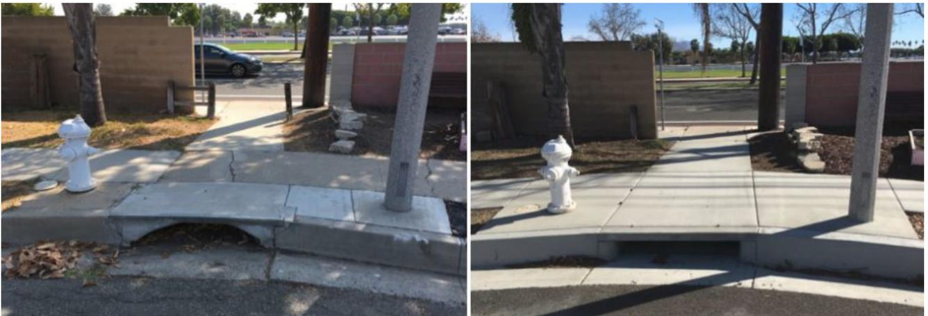
Public Services also recently completed the reconstruction of the parkway drain at Wellesley Lane near Fairview Road (see before and after photos). The project entailed demolition of the deteriorated parkway culvert and reconstruction of a parkway drain to meet the city's standards. In addition to improving drainage conditions in the cul-de-sac, the project also included minor improvements to deteriorated sidewalk to eliminate displacements.
