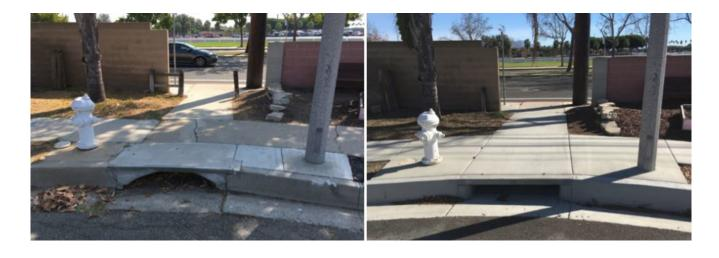
Public Services also recently completed the reconstruction of the parkway drain at Wellesley Lane near Fairview Road (see before and after photos). The project entailed demolition of the deteriorated parkway culvert and reconstruction of a parkway drain to meet the city's standards. In addition to improving drainage conditions in the cul-de-sac, the project also included minor improvements to deteriorated sidewalk to eliminate displacements.
