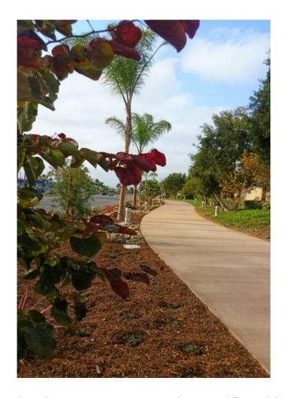
The improvements to the trail, which spans the west side of Harbor Boulevard between Fair Drive and Merrimac Way, consisted of the removal of the old asphalt trail and concrete sidewalk, and construction of a 12-foot wide, colored concrete multipurpose trail.
